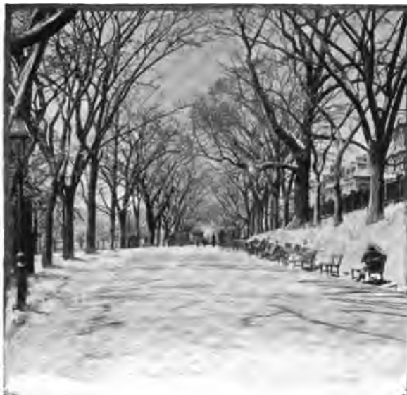
THE BEACON STREET MALL.
